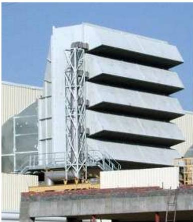
Air intake filter housing for gas turbines
