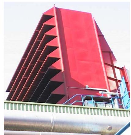
Air intake filter housing for gas turbines
